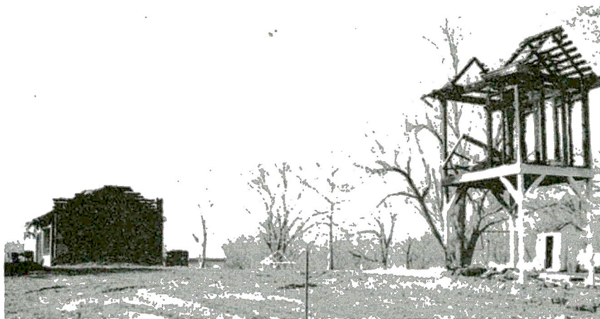
Movie site, home and racing homer loft destroyed by fire in January 1991.
